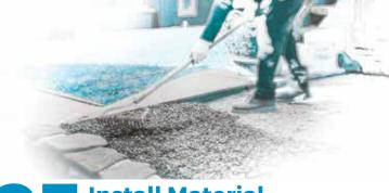
Pour blended pebble mixture directly onto subbase and rake or screed into place. EkoFlo treated pebbles should be installed within 15 minutes of mixing.
